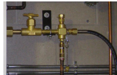
20" Header Length (Header pictured above accommodates 2 - 72" flexible pigtails for 2 portable bulk vessels, plus relief valve with pipe away)
